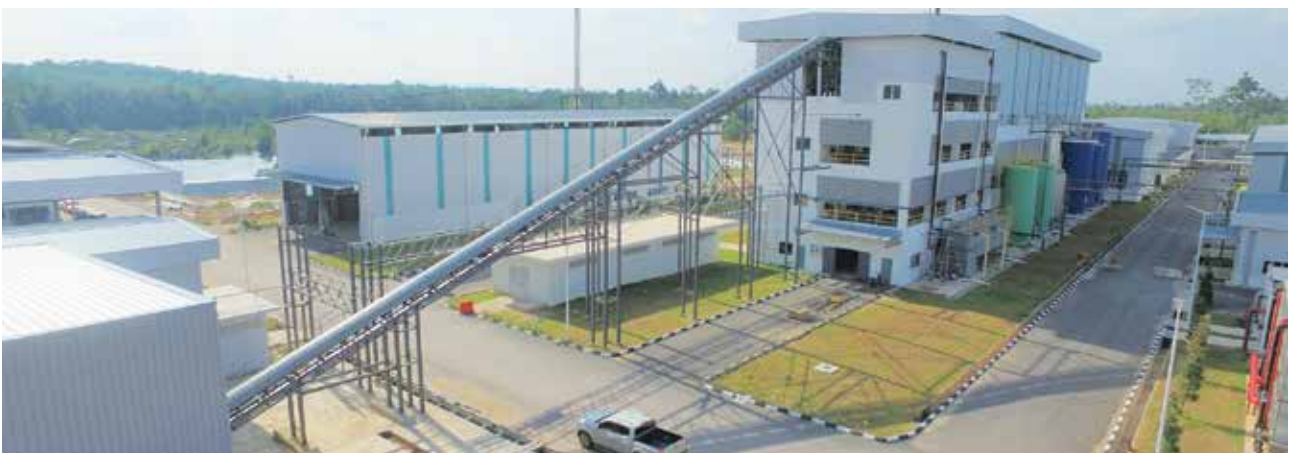
Latest photo of Phase 1A - Pulp & Paper Manufacturing Plant in GTP, Pekan.
